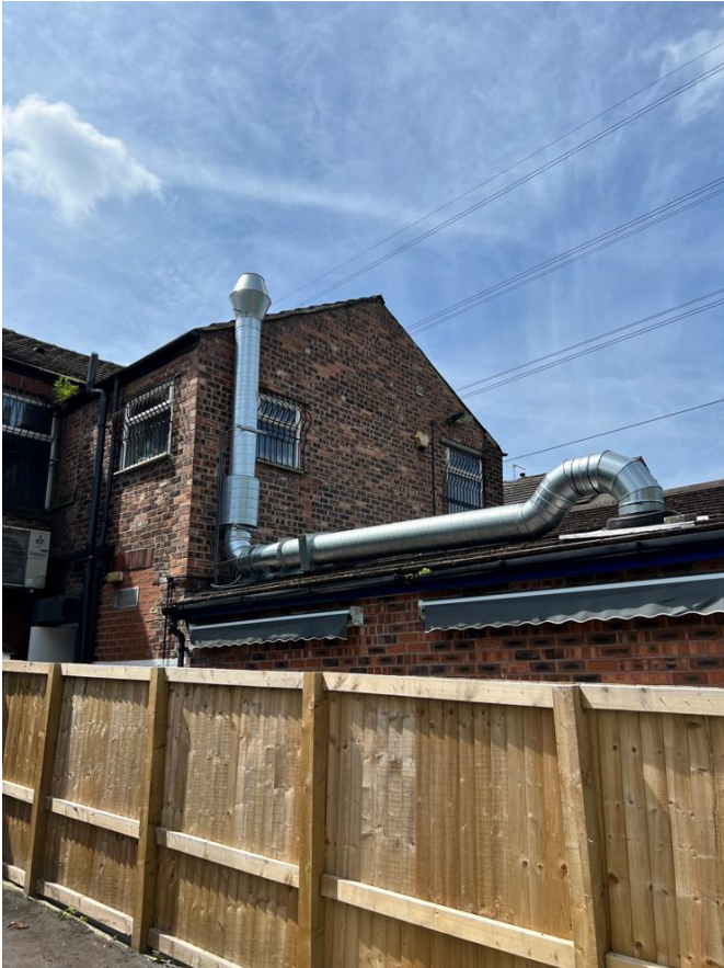
Photo 8: Extended Flue – Annotated
