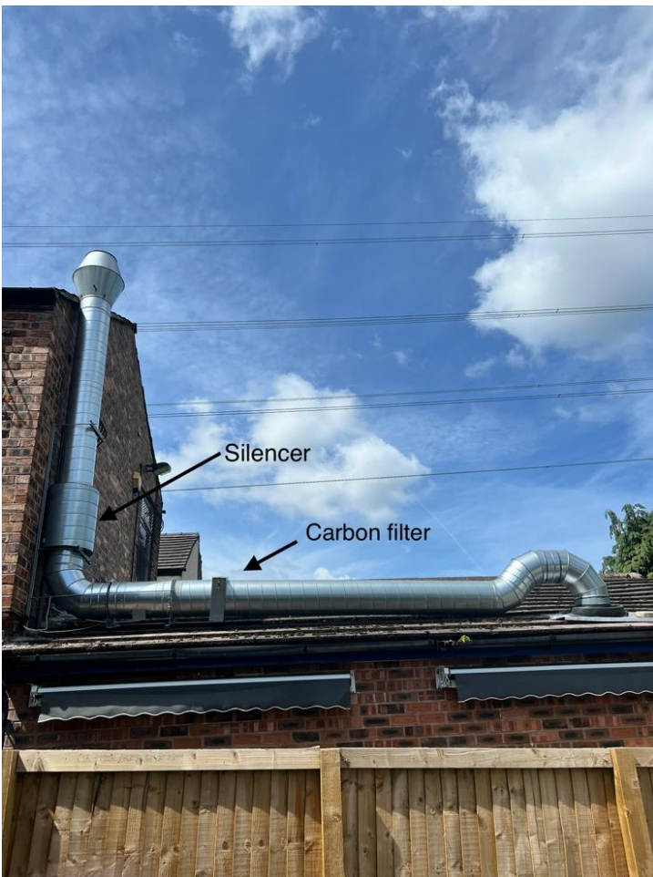
Photo 8: Extended Flue – Annotated
